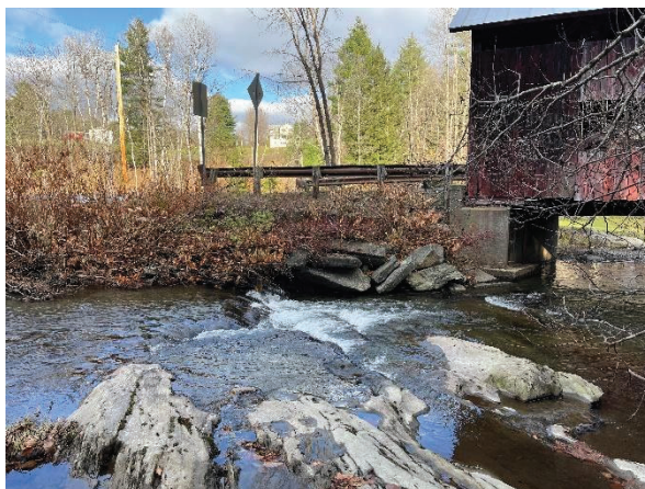
Upstream Channel with Exposed Bedrock
