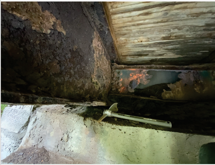
Beam 1 abutment 2 end
