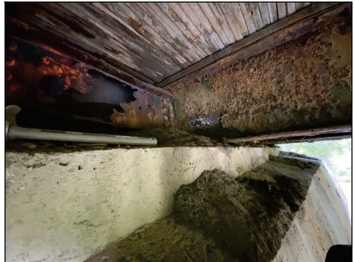
Abutment 2 beam ends
