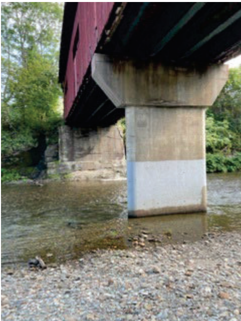
The underside of bridge 11. Taken 9/6/2023
