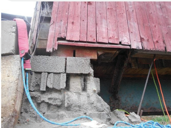
Timber Bearing and CMU Blocks
