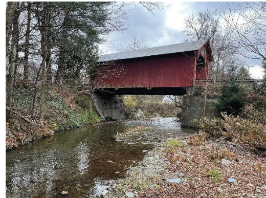
Upstream Elevation Looking South
