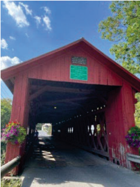
Bridge 10, taken on 9/6/2023
