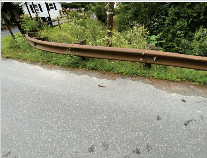
Downstream abutment 2 approach
