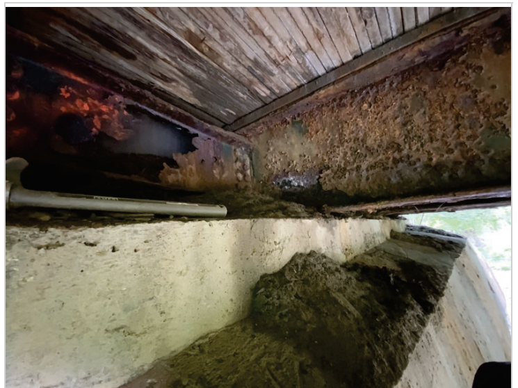
Abutment 2 beam ends
