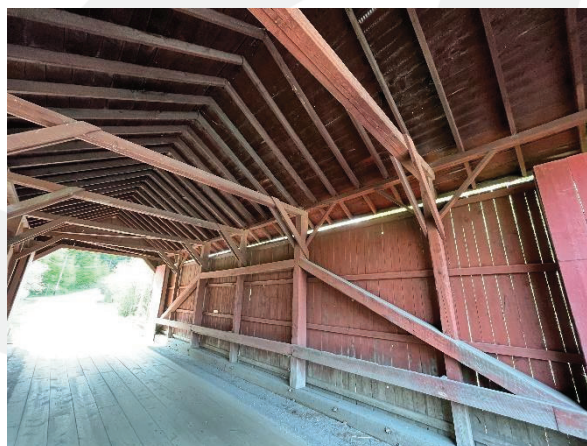
North Queenpost Truss
