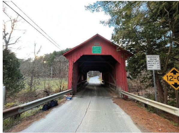
East Portal Looking West
