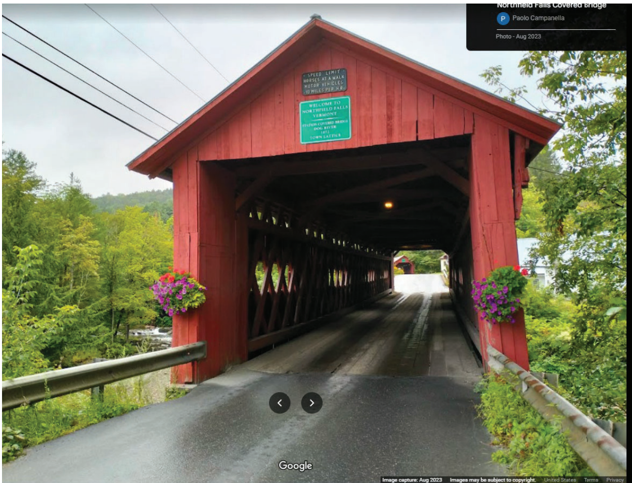
A picture of bridge 15 from google earth
