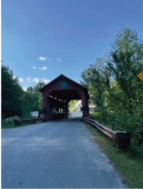
A picture of bridge 10, taken on 9/6/2023
