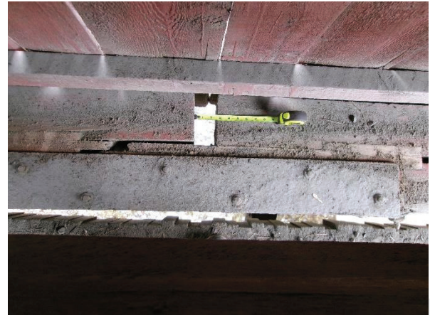
South Truss Splice at Bottom Chord
